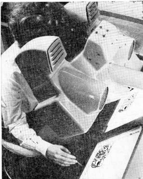
A Palmer Aero technician uses the microscope to detect possible missing holes. Using a master board, to her left, she compares it with an unchecked board. Any missing holes will flash on the viewer of the machine
