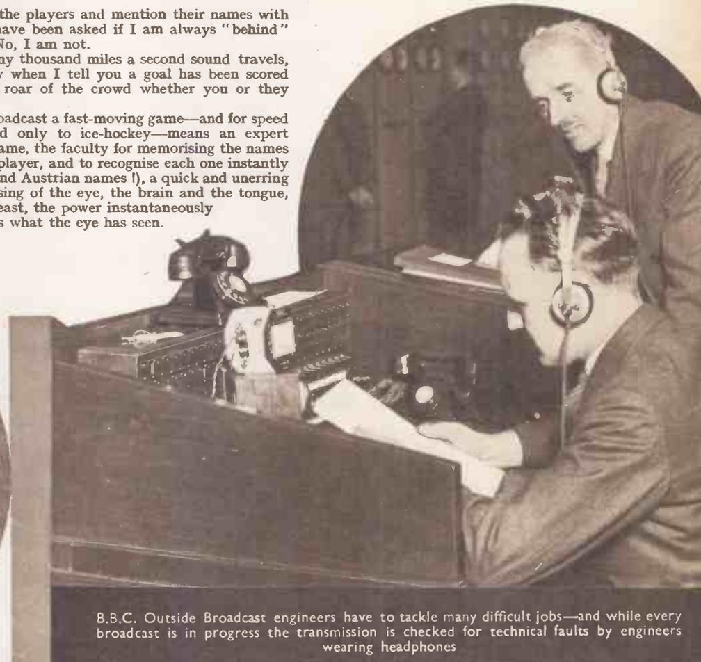
B.B.C. Outside Broadcast engineers have to tackle many difficult jobs—and while every broadcast is in progress the transmission is checked for technical faults by engineers wearing headphones
