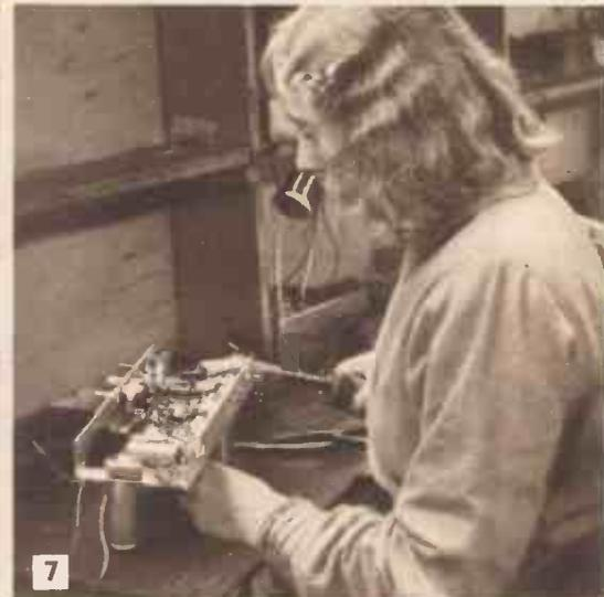
7. At this state the chassis has progressed considerably, as you can see. The volume control, wave-change switch and scale plate have all been added, together with other small condensers
