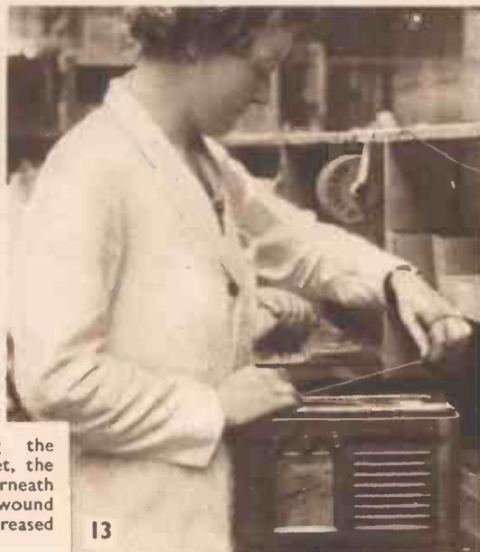
13. After screwing the chassis into its cabinet, the aerial is wound underneath—but this can be unwound and spread out for increased selectivity
