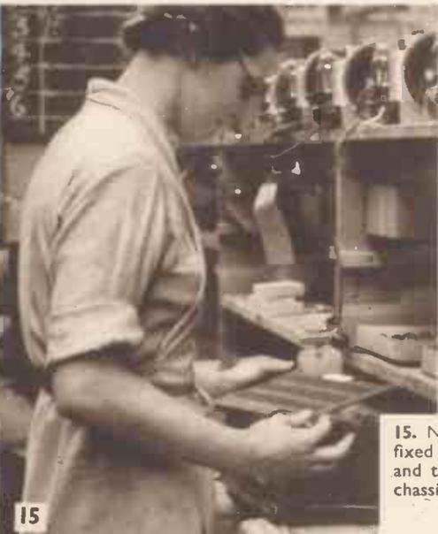
15. Now the back is fixed on the receiver, and the number of the chassis recorded for reference
