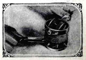
Assembling the tuning unit after all of the sections have been rewound according to the data furnished in the text.
