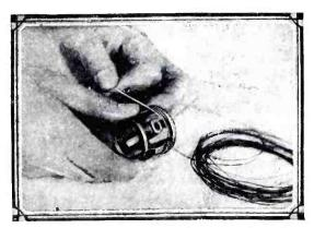
The tickler coil is rewound, using the wire that was removed from the original secondary. Twelve turns are to be used.
