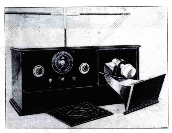
A front view of the set with the loud speaker unit and horn removed. The dial used on the shaft of the variable condenser is preferably of the vernier type in order to provide micrometer control.
