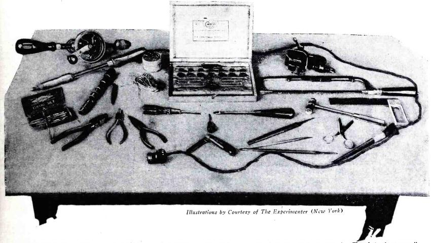
"A good worker is no better than the tools he works with." Expensive tools are not necessary, careful use of them is. The photo shows a well-selected set for the radio constructor. The set of dies and taps are not essential.
