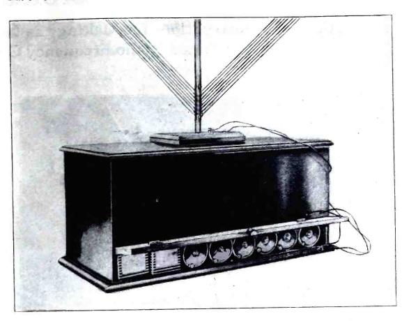
Rear view of the cabinet showing how the "A." "B" and "C" batteries are installed in a compartment. This compartment is provided with a hinged door, making the batteries easily accessible. Also note how the leads to the loop are brought out through two holes in the rear.
