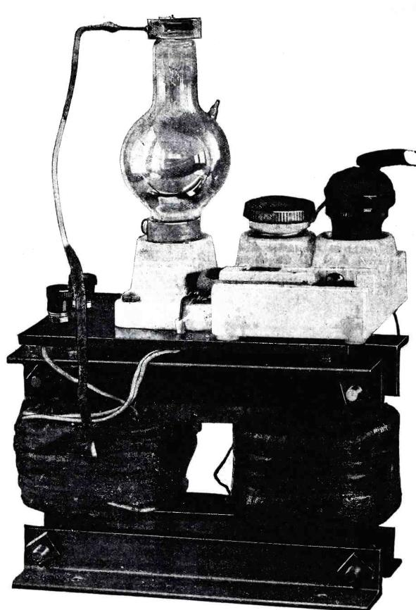
Fig. 4. How the made-up charger looks. A bakelite panel, situated above the transformer coil supports the output terminals, tungar tube, socket and input socket with fuse block.
