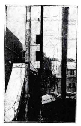
Fig. 1 (left hand photo), showing how one of the poles is held in place. This is at the slanting portion of the roof. Note the large amount of rope holding the pole. Fig. 2 (at right), showing how the pole which is at the cornice of the roof, looks. Note the guy wire coming down from the pole.
