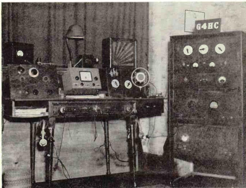
Station G4HC, Colchester, Essex. Though on a DC mains supply, AC power is obtained from a 400-watt rotary converter. The Tx is 6V6-807, the modulator uses P/P 6L6's in the output, the Rx is an HRO, and the aerial is as described in a pre-war issue of our *Short Wave Magazine*.
