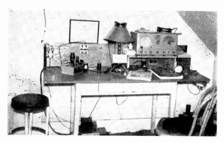
WISVL of Taunton, Mass. is one of those W's who use the simplest gear. The Tx is a 6L6-6L6 oscillator doubler and the receiver an NC-57. The station is located in an attic.
