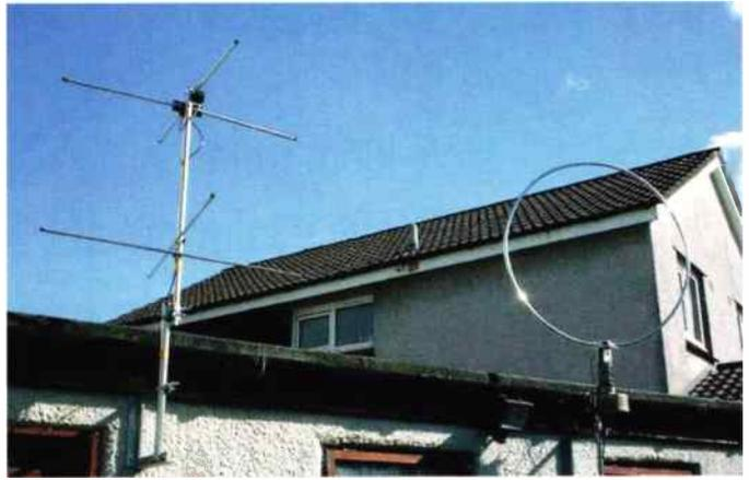
Here are Dougie's two external antennas: a turnstile for satellite work and a Wellbrook ALA1530 active antenna for h.f. There is also a long wire and a host of internal antennas mounted in the loft.
