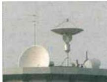
**Fig. 5: EUMETSAT's METOP dish and turnstile antennas - courtesy David Taylor.**
