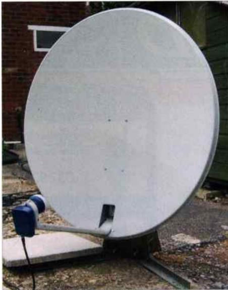
**Fig. 12: Typical METEOSAT-8 (HotBird-6) receiving system.**
