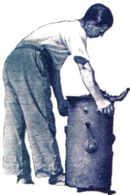
**Fig 6: Installing a Salvita III lifeboat transmitter.**
