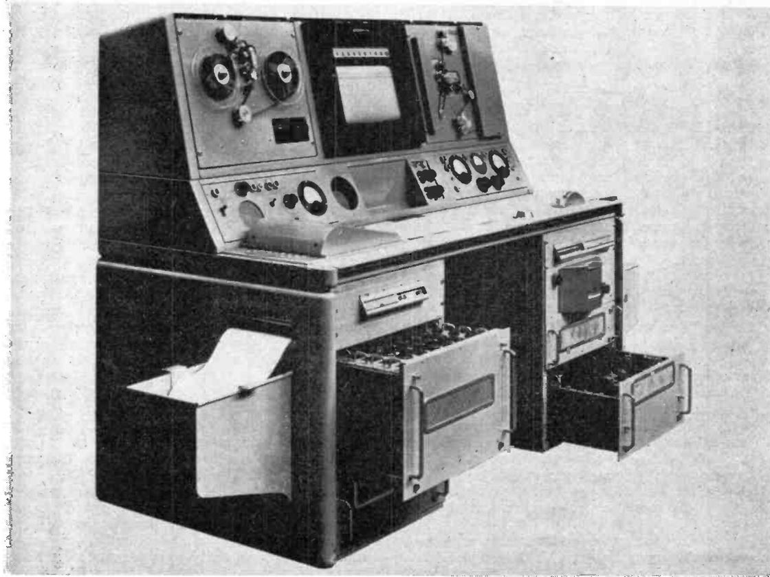
A data recorder, the Mervyn Midas, in which the usual mirror galvanometer with photo-sensitive recording paper are replaced by a tape medium. In this case, "Scotch Boy," made by Minnesota Mining & Manufacturing Co., is used. Tape recording ensures a wider frequency response, a higher system accuracy and produces a record more suitable for analysis.
