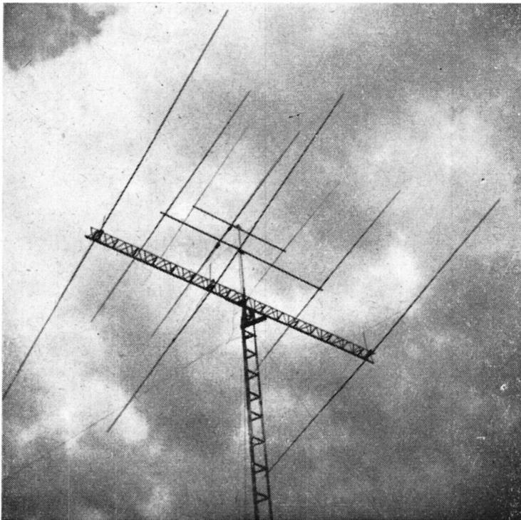
W8QGE of Detroit, Mich., has a three-band beam array, for 10, 15 and 20 metres. The tower, which is 50ft. high, is footed in a ton of concrete. All three beams are full size, and the input at the bottom end is 200 watts.
