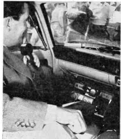
Seen at Saundersfoot, June 20. GW3MOP/M has his 160m. gear in a neat wooden case; the rig consists of a Command Rx and Codar A.T.5 Tx, easily removable for /P or fixed-station use.
