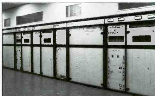
▶ 8. Now the transmitter hall contains the three transmitters, the electrical switchboard and also the special automatic monitoring equipment and computer-type controller that keeps the Regional Operations Centre in South Wales fully informed.
