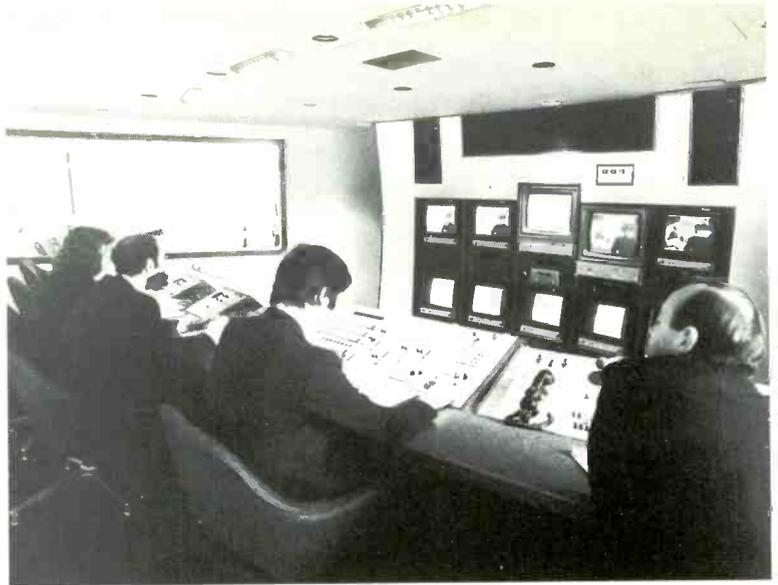
1. The vision control suite forms part of the studio production gallery. Pictures from different cameras can be selected by 'cuts' or 'mixes' or by one of many special effects. At this stage picture and sound are treated separately.
