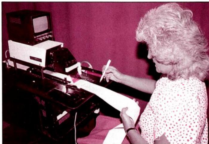
Above, Newscasters read their words using a 'teleprompter'. The script is wound through at the speed of the newscaster's voice by the teleprompter operator and appears as a reflection on specially angled glass in front of the camera's lens, visible only to the newscaster. The operator is also able to make last-minute corrections to the script. ITN
