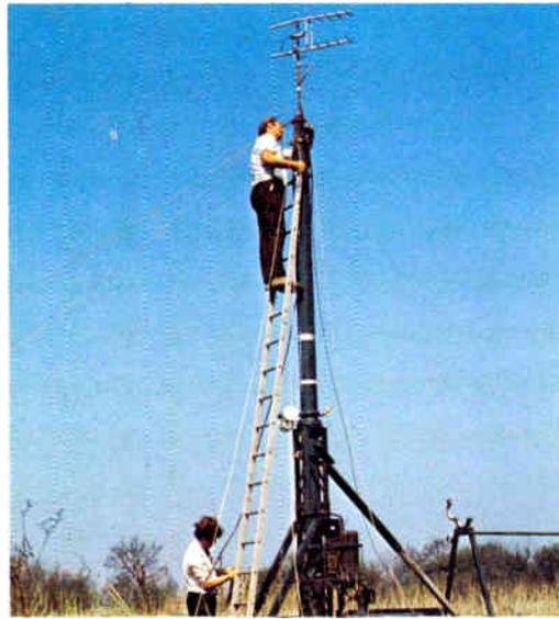
IBA engineers carry out reception tests before selecting a suitable site for a new transmitter.
