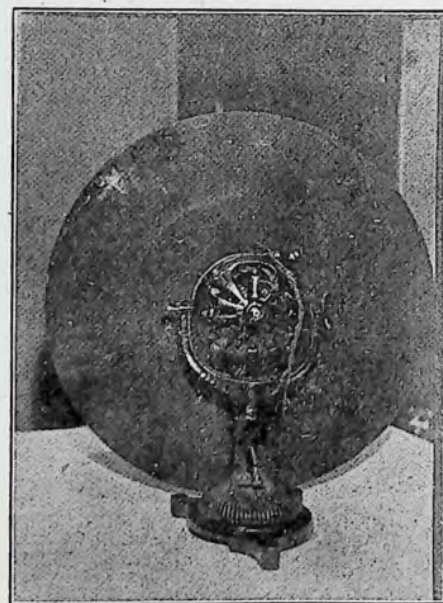
One of the scanning discs and driving motor.
