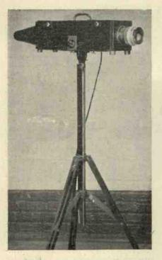
A new electron telescope with which it is possible to see through fog by means of infra-red light.
