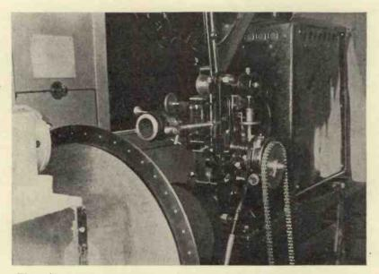
The 90-line experimental transmitter used by the International Television Corporation for test purposes. The disc and film are driven by two separate synchronous motors.
