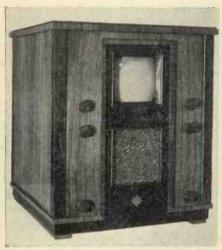
[Photo courtesy Telefunken The Telefunken 180-line cathode-ray receiver.
