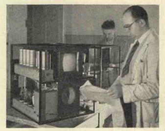
The chassis of the Telefunken cathode-ray receiver.
