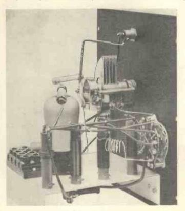
A small chassis has to be used on which to mount the components for the phone monitor and notice that the 10-metre coil is air spaced and mounted in the The wiring. remainder of the coils have a very simple fixing with one 6 B.A. bolt.
