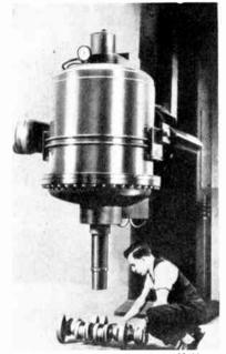
The General Electric 1,000 kV X-ray Fig. 3. tube, (Courtesy of the Victor X-ray Corporation, Ltd.)
