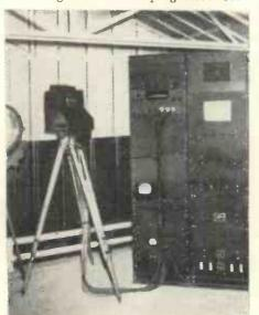
B.T.H. Iconoscope scanning equipment in the **Television Laboratory**
