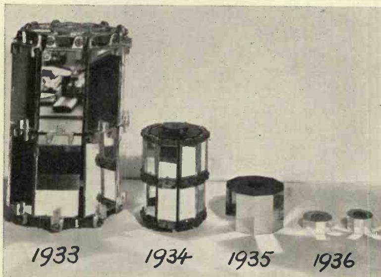
In the model we saw the 9-sided polygon is about 2 in. high and 2 in. across the faces and this for a 180-line picture revolves at 6,000 revolutions per minute, or 8,000 revolutions per minute for 240 lines.
