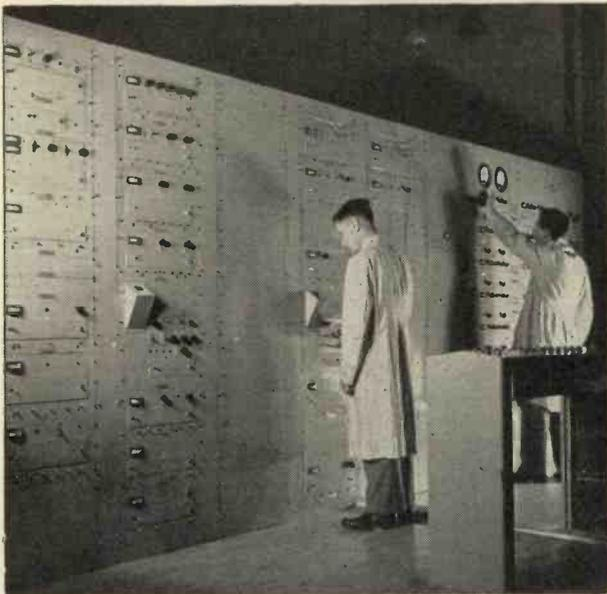
Marconi-E.M.I. control room. Emitron camera amplifiers (right), synchronising oscillators (left).
