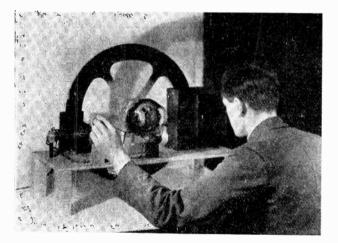
Showing how the motor is run up to speed while watching the image formation.
