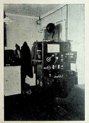
Marconi 500 watt telegraph-telephone set working on 4 10 metres (with adaptor unit for 600 metre wave working) installed at Prince Olaf Harbour, South Georgia, the most southerly wireless telephone station in the world.
