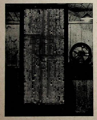
A "close-up" of the screen showing the small metal filament lamps in their honeycomb compartments.
