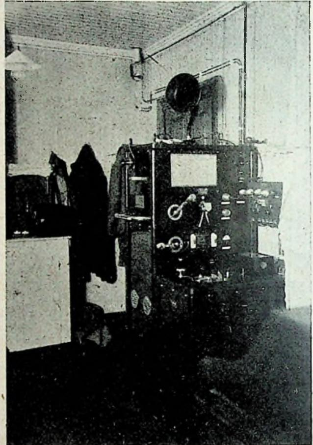
*Marconi 500 watt telegraph-telephone set working on 410 metres (with adaptor unit for 600 metre wave working) installed at Prince Olaf Harbour, South Georgia, the most southerly wireless telephone station in the world.*
