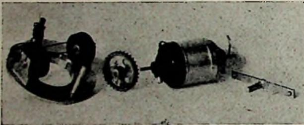
*Parts of the Baird synchronising mechanism shown dismantled from the motor.*
