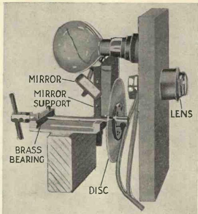
Fig. 4. A photograph of the actual chopper assembly. It will be seen that the mechanical construction is quite simple.
