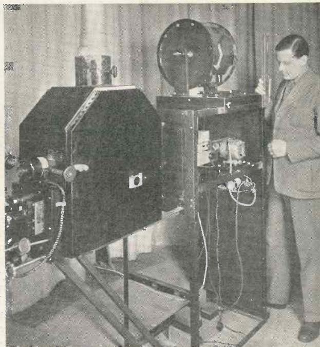
5 ft. x 4 ft. projector showing high-intensity arc, slow speed mirror drum and high-speed scanner motor. This projects a picture of considerable brightness on to a rear projection screen. The size of the apparatus can be gauged from the engineer standing at the side.
