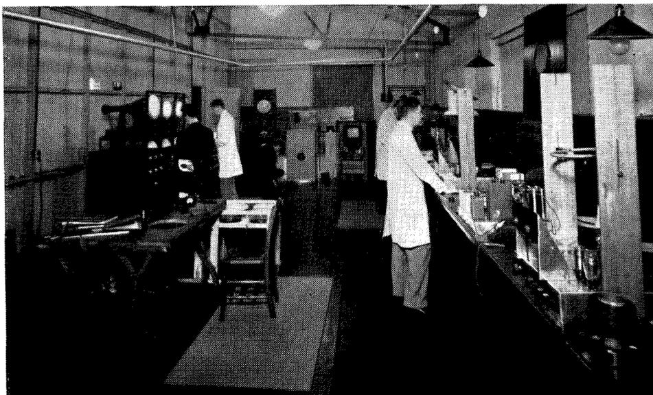
*The two test receivers are at the far end and to the left of these is a monitoring panel. On the left is the tube life test rack.*
