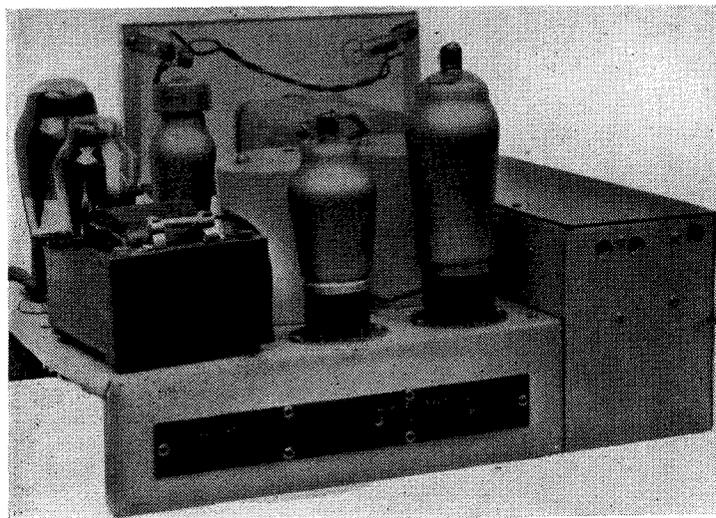
*All external connections are made to this special Clix strip which is mounted on the lip of the chassis. Padding condensers can be seen at the back of the tuner.*
