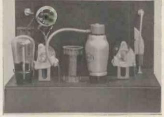
The detector and audio stages are shown in this illustration which was taken when the receiver was being used on 160 metres.
