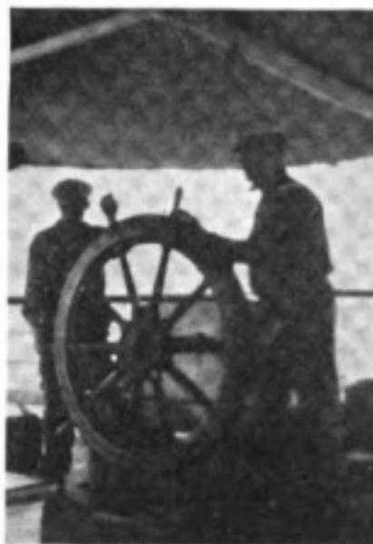
*Two "huskies" steering the Seguranca with emergency gear when the cable of the mechanism usually employed parted*
