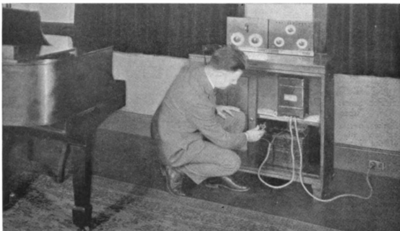
Practical installation of a Tungar outfit for charging storage batteries in the home
