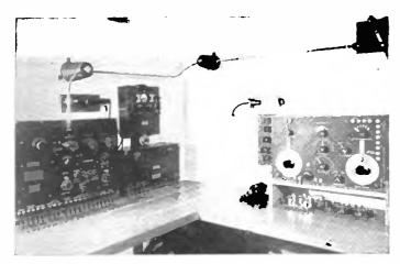
The 5-watt Western Electric C.W. transmitter and RCA, type IP-500 receiver
