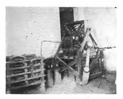
Figure 2. The antenna oscillatory transformers at the Colomb Bechar wireless station
