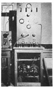
The transmitter with generator in the cabinet
