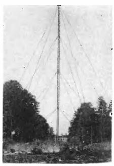
One of the towers supporting the great transmitting antenna at the new French Radio Central, located at St. Assise, near Paris
