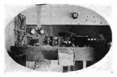
Pigure 6. The Taghit E3 bis 500-watt continuous wave transmitter equipment
