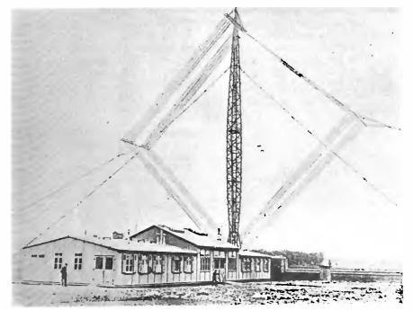
This is not a direction finder, as might be expected, but a novel form of transmitting antenna at the new German wireless station at Oranienburgarstrasse. Signals from this antenna are so strong as to be audible not only in all parts of Europe but in North America and in Asia
