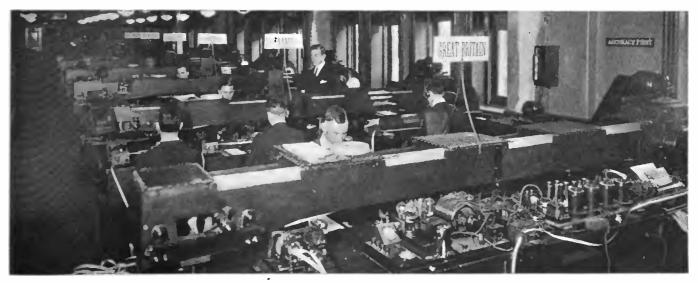
The great receiving room at 64 Broad Street hums with activity night and day, handling traffic at high speeds. Each table controls the complete circuit of a transmitter and receiver that works with a foreign country—transmitting on one side and receiving on the other. As the signs indicate, tables are devoted to service with Norway, France, Germany (2) and England (2)
