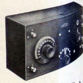
HARKO SENIOR MODEL V. A combination Tuner and Audion Detector. Equivalent to a combination of the CROSLEY CRYSTAL RECEIVER MODEL I and CROSLEY DETECTOR UNIT. one hundred miles.
