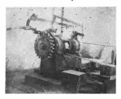
Figure 4. Belt-driven rotary spark gap of the Colomb Bechar spark transmitter
