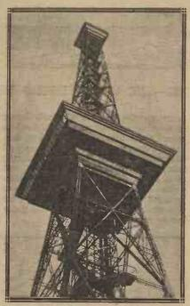
This "Radio Tower," recently erected in Berlin, is 400 feet high, and is designed for use in connection with broadcasting in Germany.
