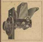
LOW LOSS—Losses minimised, the supports between the fixed and unoving plates being two only and as short as possible with very small area surface of round design.
