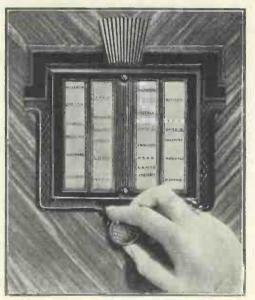
THE LATEST IN DIALS A new type of German tuning dial. As the knob is turned a light strip illuminates the name of the station to which the set is tuned
