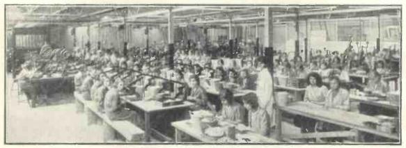
THE HOME OF THE TERMINAL AND THE WANDER PLUG Part of the main show at the Belling Lee factory. In the foreground can be seen clamping and eyeletting processes, with a power bench on the left.
