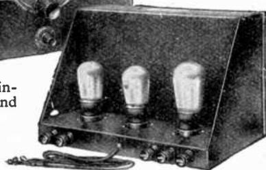
Completely enclosed—thereby eliminating dust and minimising the possibility of damage. Ready to be fitted into any cabinet or can be used without if desired. The new model is fitted with a highly efficient wave-trap, which makes tuning extremely simple.
