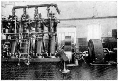
335 B.H.P. Willans Diesel Oil Engine installed at MANDALAY
