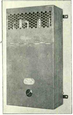
Fig. 14. Apparatus for obtaining L.T. and H.T. from A.C. mains.
