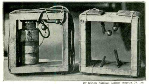
Marconi's first short wave tuned Transmitter.
