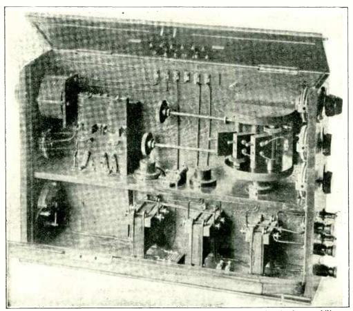
The Receiver with valves removed and coil holder transferred to the interior for portability. Fig. 7.
