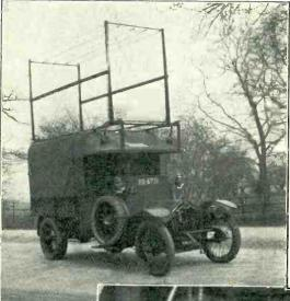
The controlling station was operated from the police headquarters in Scotland Yard, and three other wireless equipments were employed: (1) a fixed station at the race course (2) an aeroplane equipped with wireless for observing the traffic on the road and locating and reporting congested areas, and (3) a motor car equipped with wireless which could proceed to any locality on receipt of instructions from Scotland Yard and keep in touch with police patrols of motor cycles.
