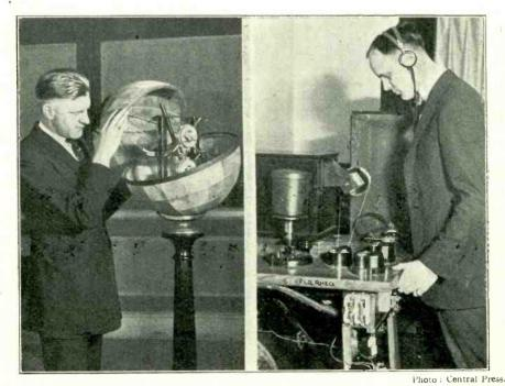
This new microphone, shown on the left, is arranged to operate the two stations WJZ and WJY. The right-hand illustration is a device for visibly indicating the degree and quality of the modulation.
