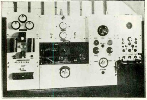
Fig. 18. The transmitting equipment of the German broadcasting station at Königswusterhausen.
