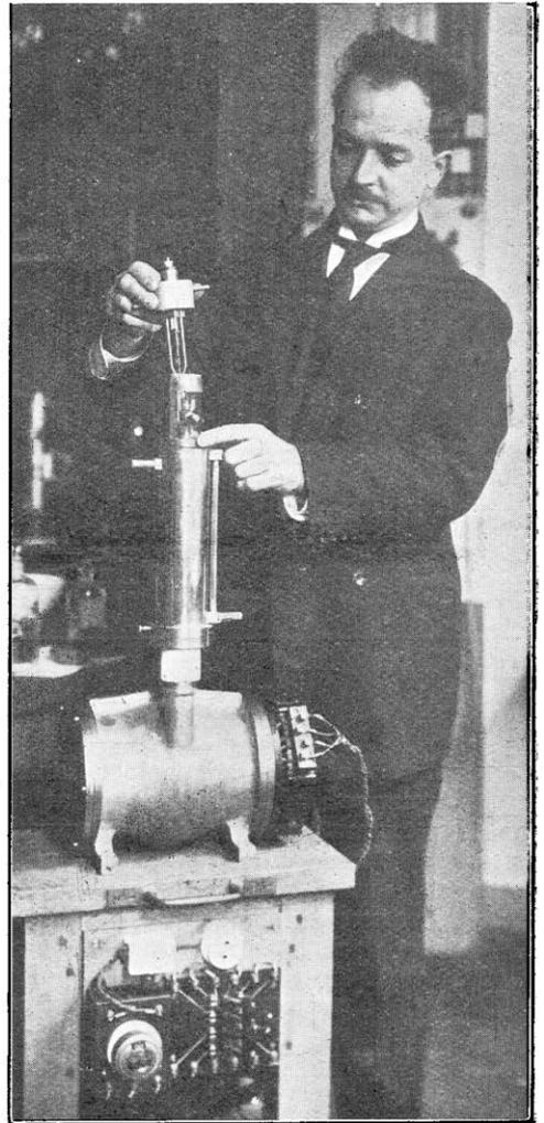
*Dr. Holweck assembling a valve. The lower chamber is the rotary pump.*
