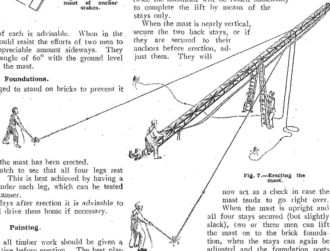
Fig. 7.—Erecting the mast.
