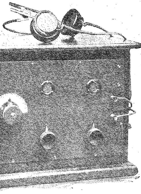
The two-valve receiver described here is a most useful set because it has only two tuning controls, and may be used for the reception of long wavelength signals as well as the broadcast by putting the appropriate tuning coils in the two-coil holder. It is suitable for telephony and telegraphy, and, as reaction is employed, is sensitive and selective. The design has been made as simple as possible consistent with effectiveness.
