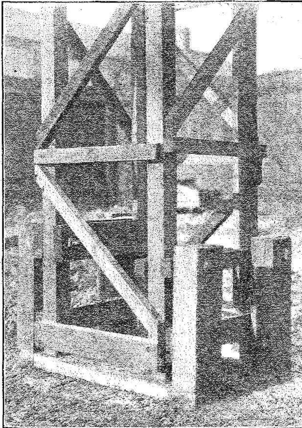
The base stands upon a brickwork foundation, and is held in position by four foundation posts.
