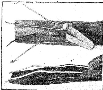
The paper supported wires used in the construction of "Cosmos" coils.
