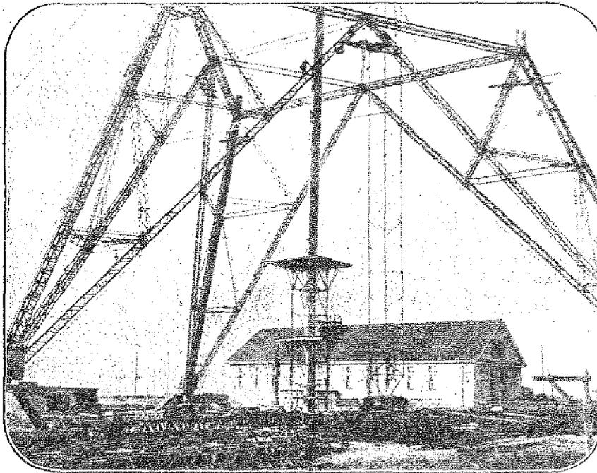
MONSTER WIRELESS MAST. Erecting the 830-foot mast at Koenigswaterhausen, which, it is stated, will be the world's largest wireless station. One of the transmitting houses is seen in the background.
