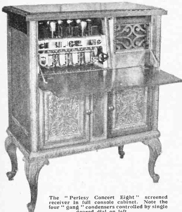
The "Perlesy Concert Eight" screened receiver in full console cabinet. Note the four "gang" condensers controlled by single geared dial on left.
