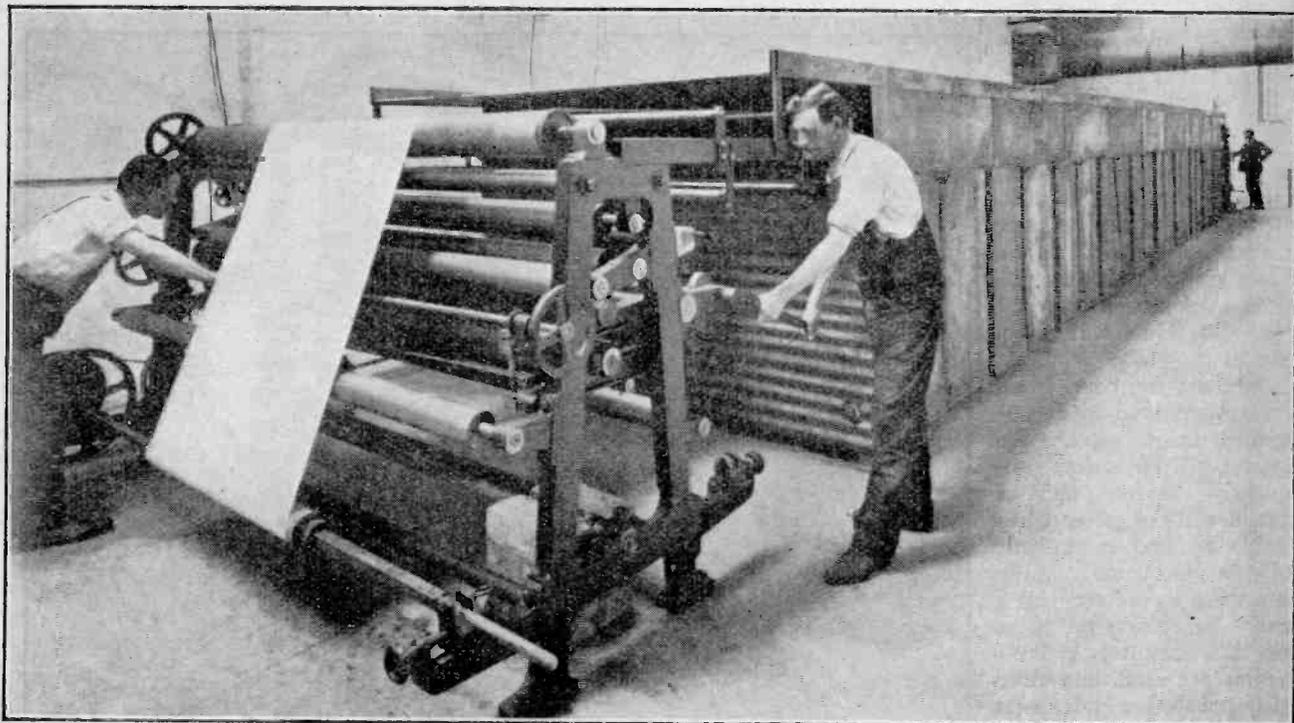
Fig. 3.—Paxolin paper varnishing machine equipped with steam-heated oven 75ft. long.
