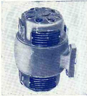
(c) Rotary Converter, Type 'C', rating 800 to 1000 watts, for use in radio sets. Can be supplied for any intermediate voltage with correspondingly lower output. Price £23 10s. 0d. including starter and enclosed heavy duty Transformer for output Voltage regulation. Approximate weight of converter, 150 lb.
