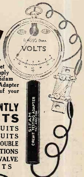
Every efficiency test of a radio set can be made simply by plugging a Sifam Circuit Testing Adapter on to the spike of your voltmeter.
