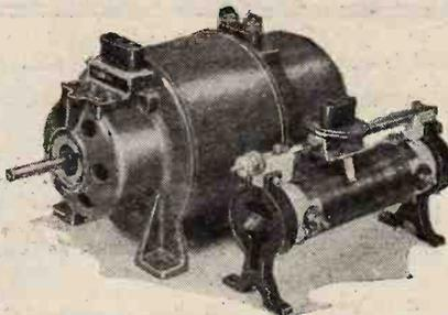
M-L rotary transformer, Type H.F.A., rated at 85 V.A. output and regulating resistance.
