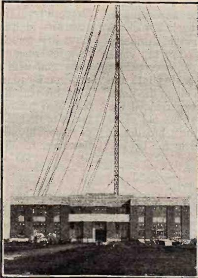
**MOORSIDE EDGE.** A photograph taken last week showing the newly completed station building for the Northern Regional transmitter. The design is identical with that of Brookmans Park. The masts are 500 feet high.
