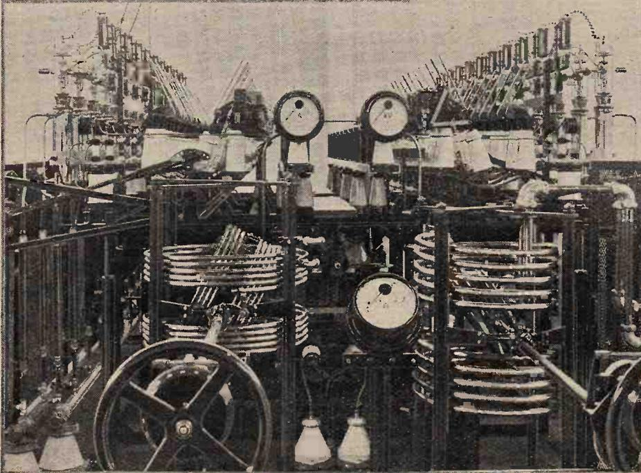
Unlike Brookmans Park station, Muhlacker does not generate its own power. All current is drawn from the local mains, a rotary converter changing the 50 cycle A.C. 15,000 volts supply to direct current for the anodes.
