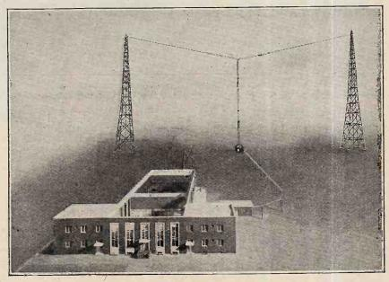
ANOTHER GERMAN GIANT. A model of the new high-power broadcasting station which opens to-day (Wednesday) at Heilsberg, Eastern Prussia, working on a wavelength of 276 metres and a power of 75 kilowatts. Like its companion station at Mühlacker, the new station can increase its output to 120 kilowatts.
