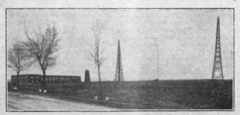
HEILSBERG. A comprehensive view of a typical German high-power station, of which there will be nine in the proposed new broadcasting scheme. The long, low transmitter house resembles the station building at Brookmans Park. The water-cooling tower and low-voltage feeder wires can be clearly seen.
