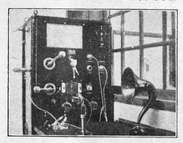
A wireless telephone set at the Post Office station at the Humber, used for communicating with fishing craft, etc.
