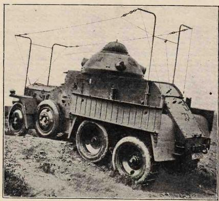
ARMOURED CAR WIRELESS. The latest type of travelling fort in use by the R.A.F. The wireless aerial is carried on collapsible metal masts.
