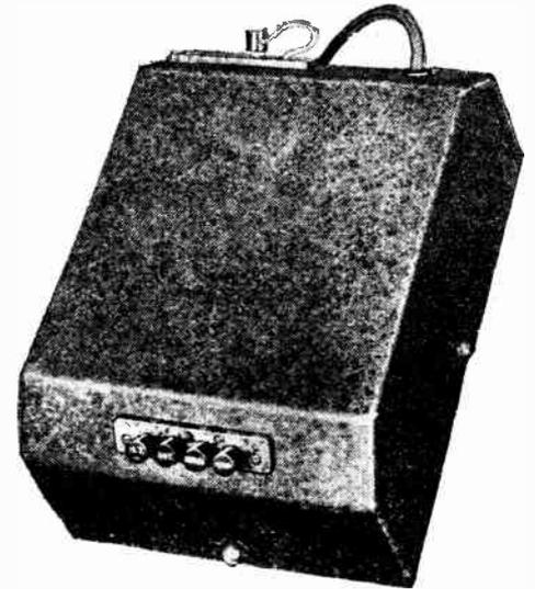
Rectifiers "Q" 20 model H.T. battery eliminator giving a maximum output of 20 mA. at 135 volts.
