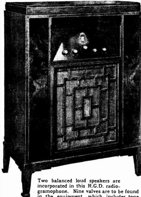
Two balanced loud speakers are incorporated in this R.G.D. radio-gramophone. Nine valves are to be found in the equipment, which includes tone control and a volume control effective on both radio and gramophone.
