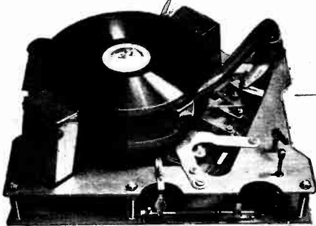
Record-changing mechanism fitted to current H.M.V. radio-gramophone.
