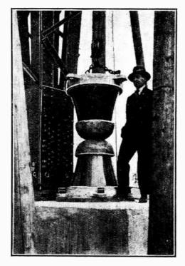
AT BUDAPEST. The base of the 1,020-ft. cigar-shaped mast of Hungary's new 120 kW. transmitter. The porcelain base supports a weight of 480 tons.
