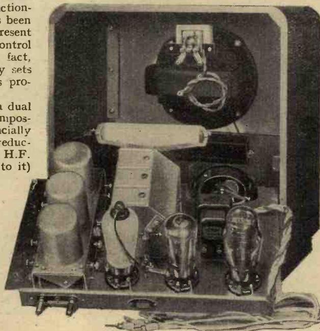
The Lissen kit set is assembled on a ready-drilled metal chassis.
