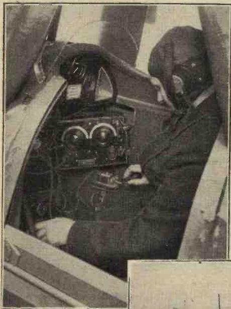
For direct communication with headquarters from the Scotland Yard Autogiro there has been installed a Marconi transmitting and receiving equipment.
