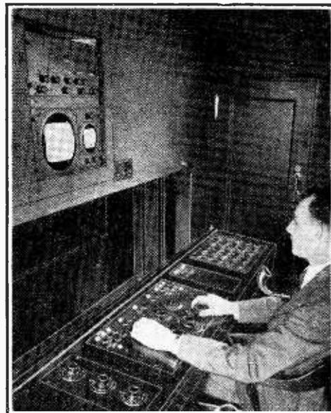
THE VISION MONITOR. Television Control Engineer at the N.B.C. Studio in New York. He controls the outgoing vision transmission and is in direct telephonic communication with the camera operator.
