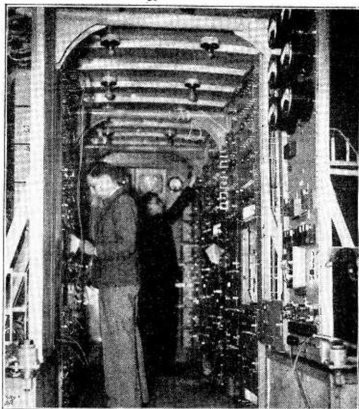
TELEVISION NERVE CENTRE. The interior of the control van which was used for the television broadcast of the Coronation Procession. At the far end of the van can be seen the two monitoring tubes on which the control engineer sees the picture as transmitted. Each tube is connected to a separate camera.
