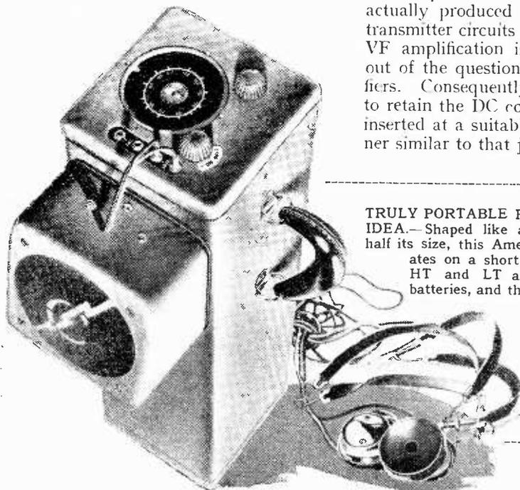
**TRULY PORTABLE RECEIVERS: A NEW IDEA.**—Shaped like a golf bag, but about half its size, this American Crosley set operates on a short trailing aerial. Both HT and LT are obtained from dry batteries, and the total weight is given as 18 lb. The circuit employs five valves, plus a barretter which presumably provides automatic regulation of filament current in spite of voltage variations.
