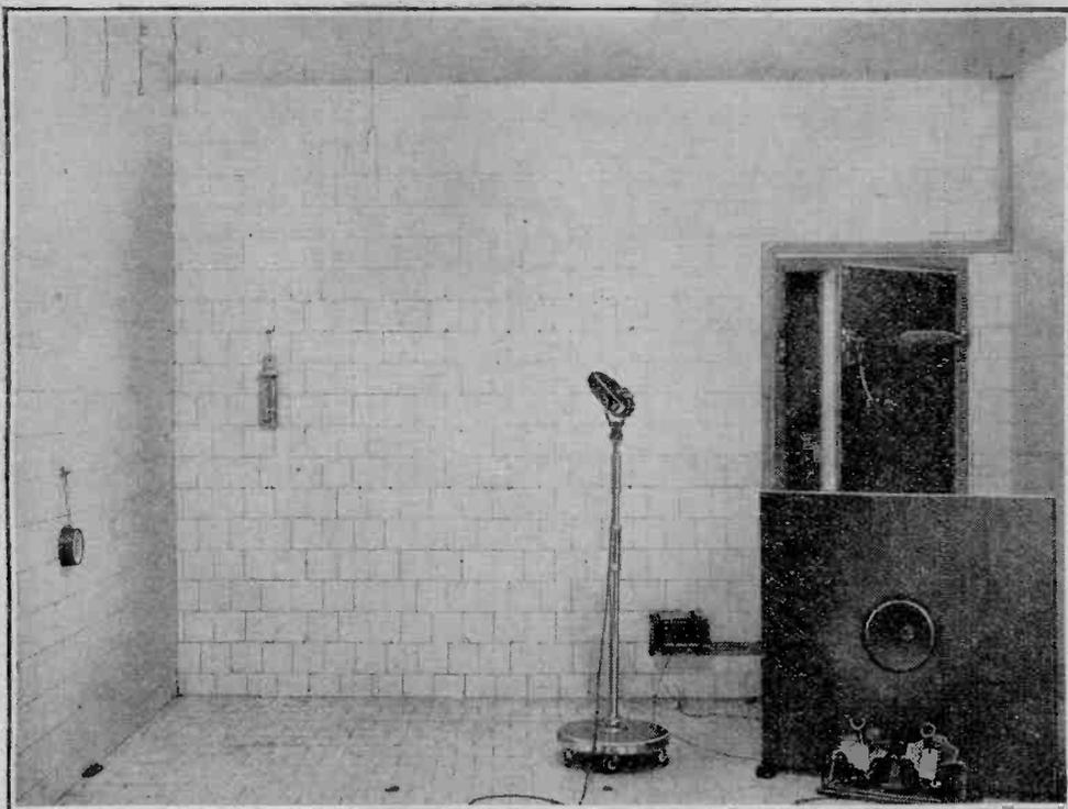
The reverberation chamber, showing loud speakers and microphone. Note the thick, sound-proof door.
